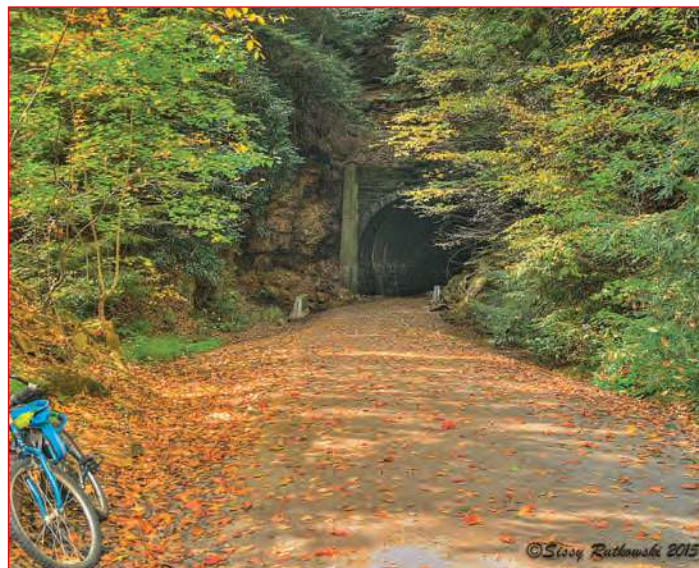
The Climax Tunnel sits along the Redbank Valley Rail Trail. Photo Credit: Sissy Rutkowski
