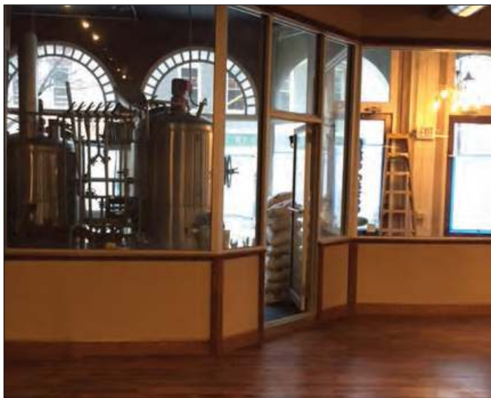
Renovations have already begun at the Blue Canoe Brewery.
